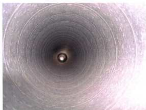
Cleaned duct level below indication of quantity
